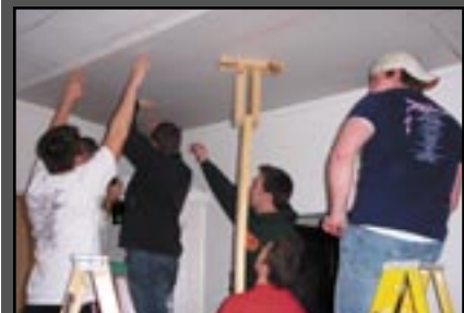
Katrina house renovation
